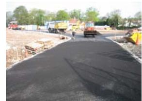
To advance the development programme, UR delivered the site infrastructure to first stage, in parallel with the remediation works, stabilising road formations to mitigate the need for well pointing during drainage installation.
