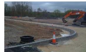
The developer's surface water drainage design conflicted with the existing foul system. Constrained by the site topography and practical pipeline gradients, the UR team provided a unique flume alternative, approved by the adopting authority and installed under running sand conditions.
