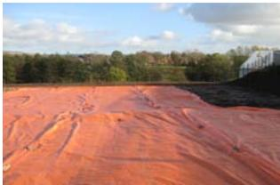
To provide a development platform for the 85 piled low cost residential properties, the below ground structures and poor quality ground required re-engineering and processing on site prior to the installation of an 800mm validated cover system in advance of the deposition of topsoil / subsoil to garden and play areas.
