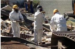
The remediation of this former mill site in Rochdale was part funded by Rochdale MBC in conjunction with Base Regeneration LLP and Barratt Homes. Advance investigation identified widespread asbestos contamination throughout the ground and significant physical substructures within the 3m+ layer of made ground consisting of hardcore and demolition rubble.
