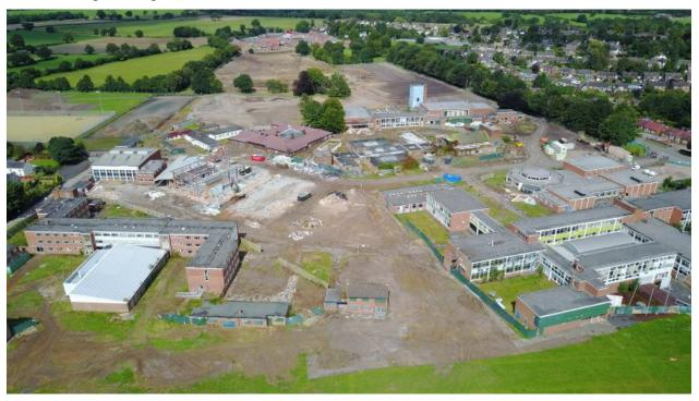
The 36-week agreed programme and consisted of significant asbestos removal, soft strip demolition, materials processing and earthworks, including the treatment of large volumes of deep made ground in discreet areas of the site.
