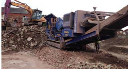
Extensive material reprocessing using our own equipment was undertaken in accordance with the CL:AIRE Code of Practice to optimise the sustainable re-use of site won materials in compliance with the Environmental Permitting Regulations 2010.
