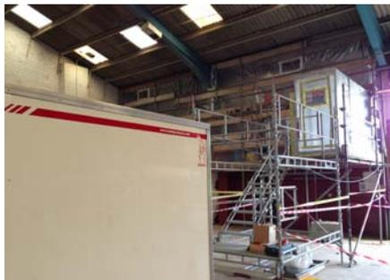
The industrial units were subjected to licenced asbestos removal and full enclosure conditions, with environmental air monitoring to verify the adequacy of safety measures to mitigate the risk to site personnel and adjacent residents.
