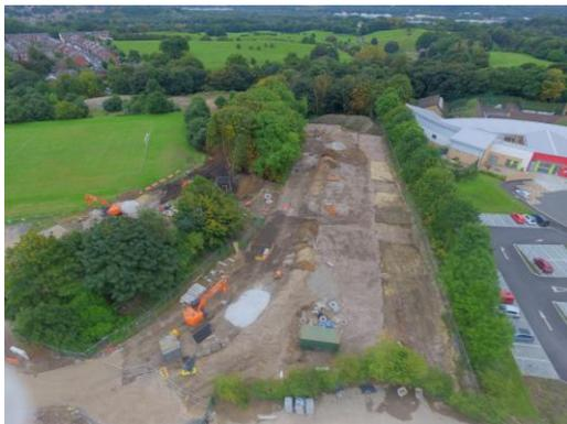
The strategy called for the segregation and set aside of sufficient topsoils and subsoils for the development, re-engineering of the site wide fills to facilitate a 50/50 vibro/piled foundation solution, the onsite relocation of knotweed to a treatment area off the development footprint, chemical treatment of invasive weed outside the immediate development area and a full re-profile of the landform through the wettest winter period Nov 2015 / Jan 2016, since records began.
