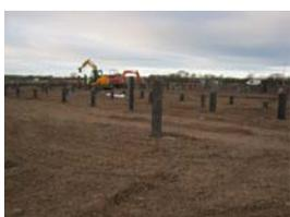
Site wide settlement monitoring was undertaken to verify the levels of consolidation within the weaker soils and were within design parameters and to the satisfaction of the NHBC. The works also incorporated recovery of large volumes of historic foundations for re-processing on site and use within the site infrastructure and the chemical treatment of over an acre of Giant Hogweed.
